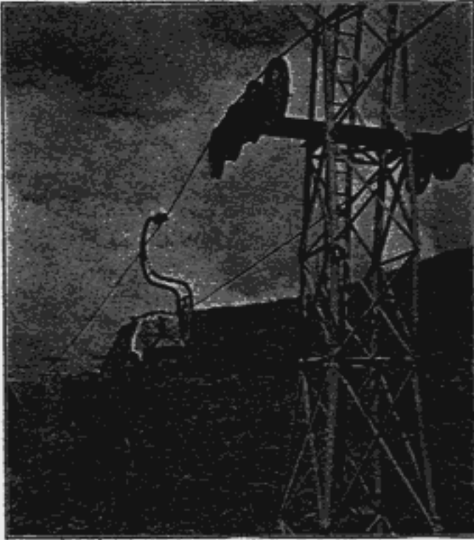
AERIAL CABLE-WAY FROM MANIZALES TO THE HONDA RAILWAY
