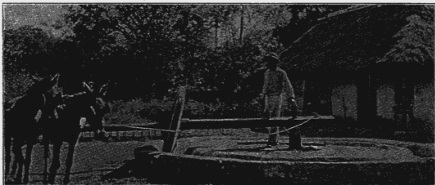
A MULE-POWER COFFEE HULLER, HAITI
